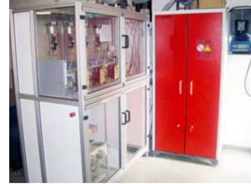
Solar cell supplied fuel cell facility with electrolysis
